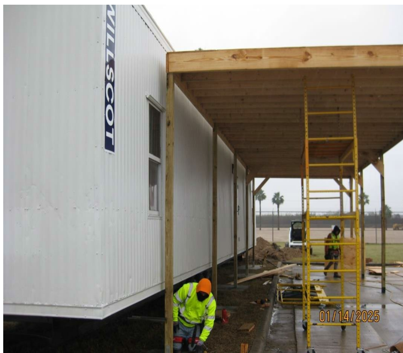
TEMPORARY OFFICE TRAILER POSITIONED AND LEVELED NEXT TO THE CANOPY
