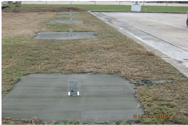
CONCRETE POUR OF THE EXCAVATED FIVE (5 EACH) CANOPY FOUNDATION FOOTINGS
