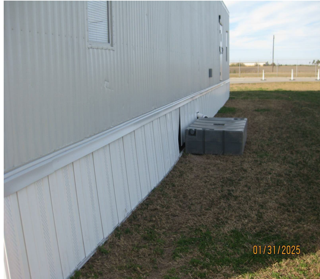
TEMPORARY BUILDING SKIRTING INSTALLED
