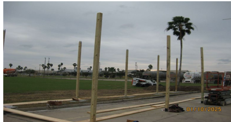
ZIWA BEGAN CANOPY CONSTRUCTION PLACING OF VERTICAL AND HORIZONTAL FRAMING
