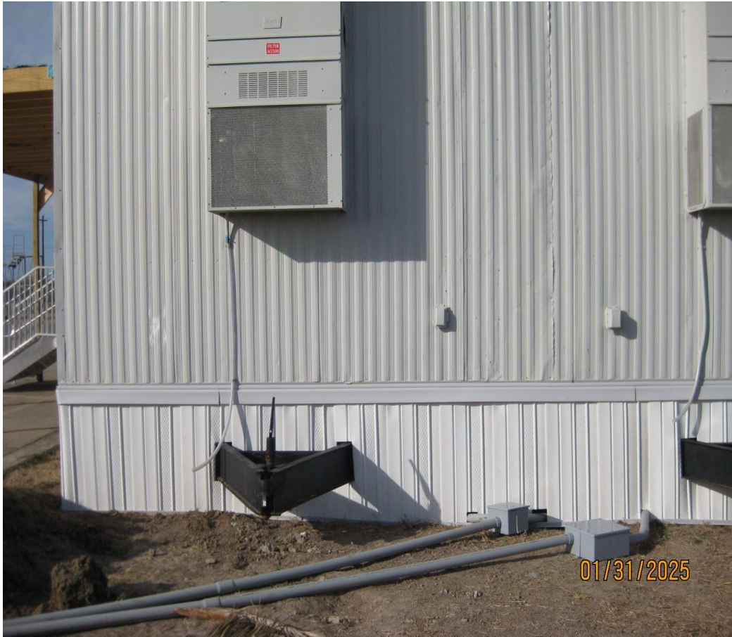
TEMPORARY BUILDING SKIRTING INSTALLED
