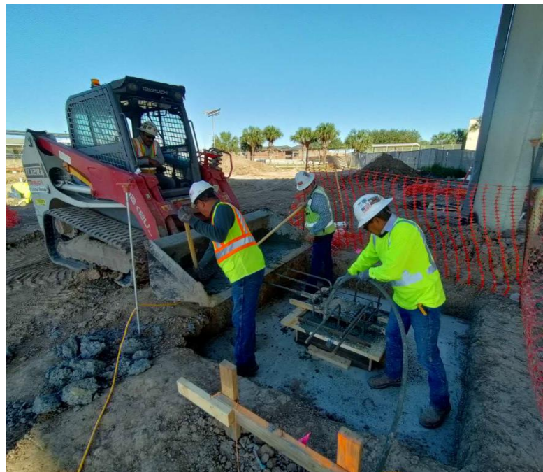
Certified Placers Tied "D" Bars onto the Footing Stem and SpawGlass Poured Concrete in the Headhouse's Column Spread Footing Stem.
