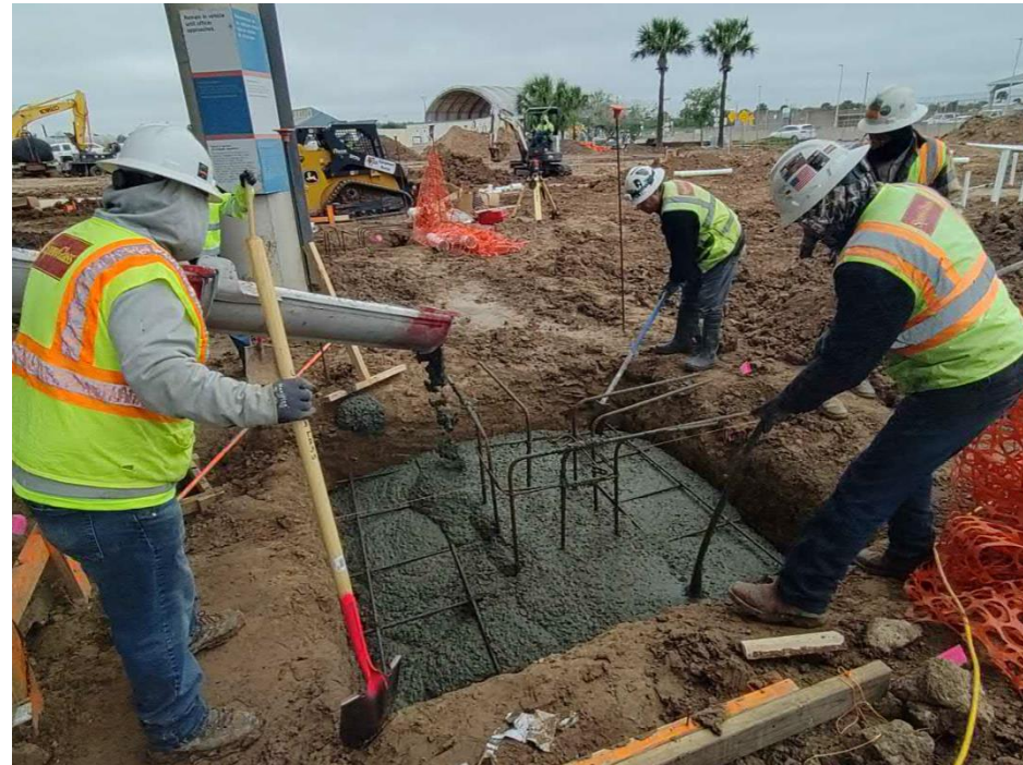
Certified Placers Tied Rebar for the Proposed Spread Footings and SpawGlass Poured Concrete into Spread Footing
