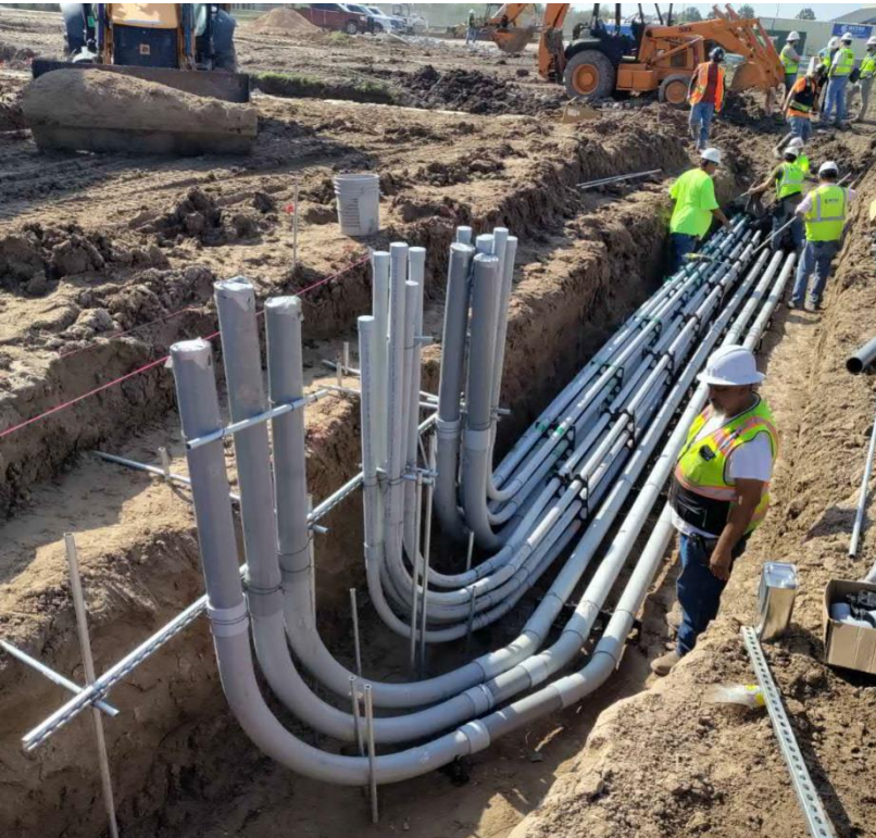
Metro Electric Placing of Communication Duct Bank Conduits
