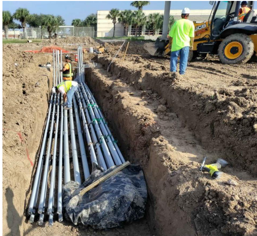
Metro Electric Placing of Communication Duct Bank Conduits
