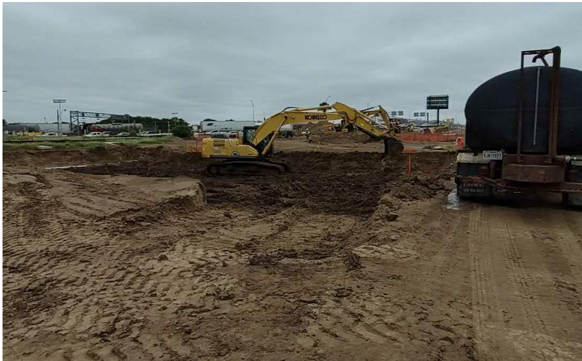
D&J Site Construction, LLC. Proposed Booth Area Excavation, Proof Rolled, and Compaction of Moist Selected Fill Material in 6-inch Lifts
