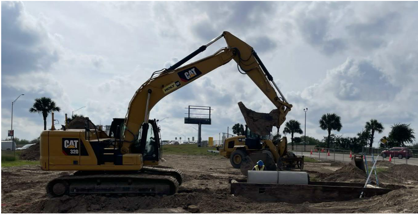
RM Walsdorf Placement and Backfill of 24-inch RCP
