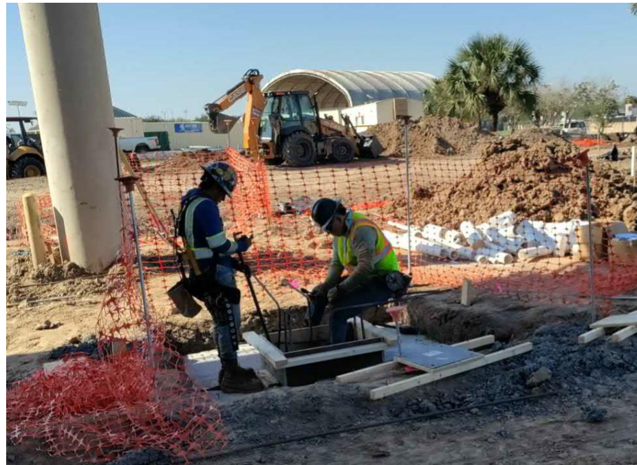
SpawGlass Formed Headhouse's Column Spread Footing.
