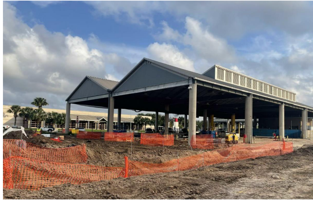
SpawGlass Excavated for Spread Footings of Proposed Headhouse
