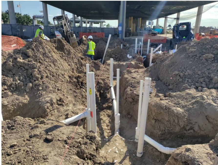
Farrell Plumbers Installation of Sanitary Sewer PVC Pipe, Backfilled with Selected Fill Material, and Compaction of the Trench
