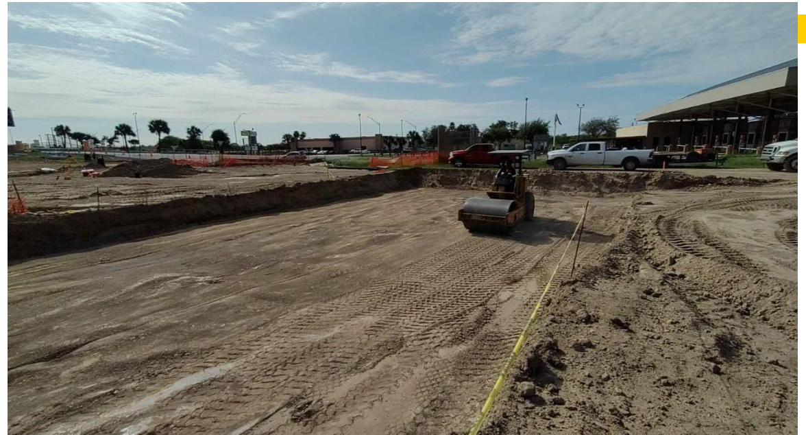
D&J Site Construction, LLC. Proposed Booth Area Excavation, Proof Rolled, and Compaction of Moist Selected Fill Material in 6-inch Lifts
