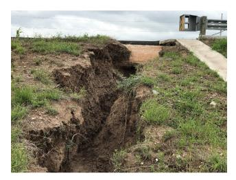
G8: Run Off Erosion at Front Slope – SBML North of FM 1847
