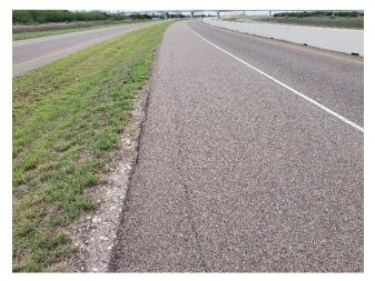
PV35: Crack in Asphalt – SBML East of Old Port Isabel Rd
