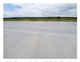
PV14: Transverse Cracking – NBML W of Ditch No. 3
