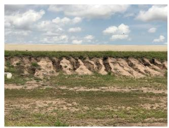
G5: Run Off Erosion at Front Slope – SBML North of RR Crossing No. 1
