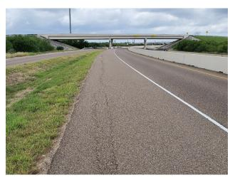
PV36: Cracks in Asphalt – SBML East of FM 511
