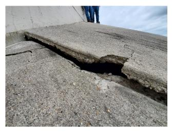
B13: Erosion Beneath Rip Rap: SBML FM 1847 Bridge
