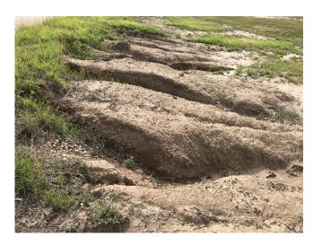
G2 Run Off Erosion at Front Slope-SBML North of RR Crossing No. 1
