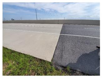
PV29: Cracking at Transition of Pavement Types – SBML W of RR Bridge
