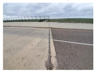
B3: Bridge Joint Requiring Cleaning and Resealing – SBML W Side of RR Bride
