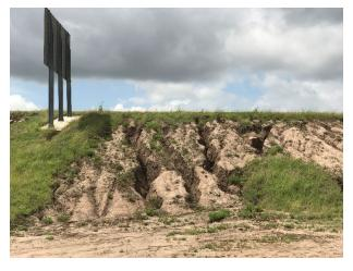
G7: Run Eff Erosion at Front Slope – NBML North of RR Crossing No. 1
