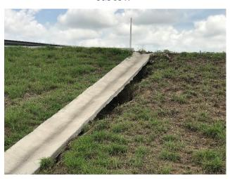
G16: Run Off Erosion Created Void Under Flume – SBML South of FM 1847
