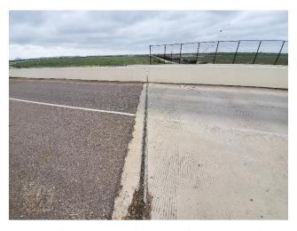
B1: Bridge Joint Requiring Cleaning and Resealing – SBML E Side of RR Bridge
