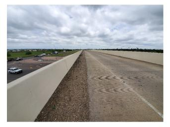
B6: Debris on Bridge Deck - SBML 3248 Bridge
