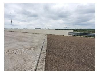
B12: Bridge Joint Requiring Clearing and Resealing – SBML W Side of FM 1847 Bridge
