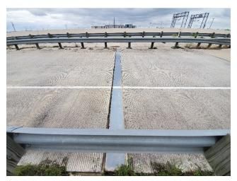
PV27: Joint Requiring Sealing & Cleaning – SBML 1st Exit Toll Gantry
