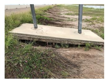
G1: Sign Riprap Exposed Due to Erosion – SBML South of RR Crossing No. 1
