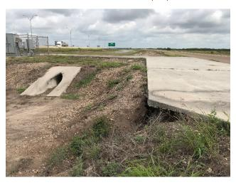
G18: Run Off Erosion Creating a Void Under Concrete Pad – NBML Toll Gantry No. 1
