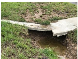
G14: Run Off Erosion Created Void Under Flume – NMBL North of RR Crossing No. 3
