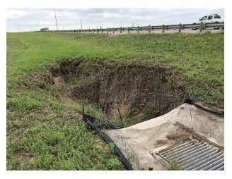
G12 Sinkhole Next to Drain Inlet – Inside Median North of Troll Gantry No. 2
