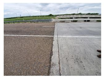
B18: Bridge Joint Requiring Cleaning and Resealing – SBML E side of Ditch No. 3
