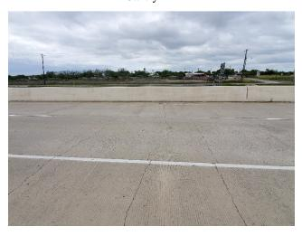
PV23: Transverse Cracking – SBML E of Entry Toll Gantry
