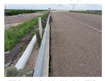
PV8: Separation of Asphalt and Mow Strip – NBML W of FM 1847
