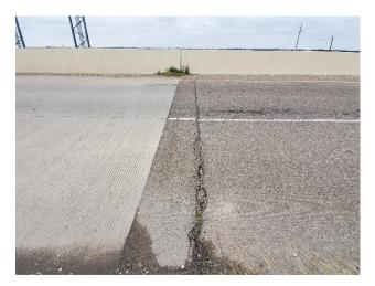
PV1: Cracking - NBML N Side of Entry Toll Gantry
