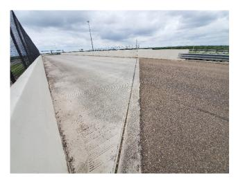
B15: Bridge Joint Requiring Cleaning and Resealing SBML W Side of 2nd RR Bridge
