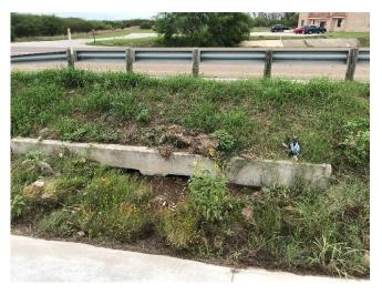
D6: Silt Accumulation at Culvert Crossing – NBFR North of Ditch No. 3
