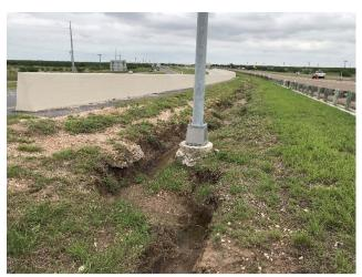
G13: Run Off Erosion Cutting Through Inside Median – NBML North of RR Crossing No. 3
