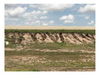
G5: Run Off Erosion at Front Slope – SBML North of RR Crossing No. 1
