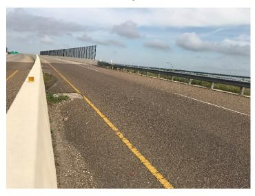
PM5: Faded Pavement Markings at Bridge Approach – NBML South of RR Crossing No. 1
