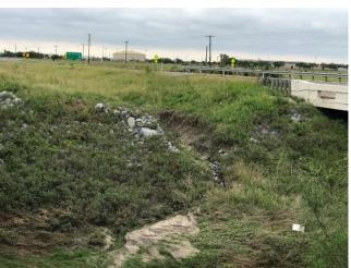
D5: Stone Rip Rap Failure – Ditch No. 3
