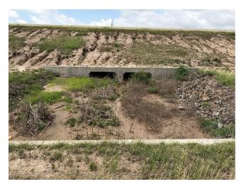
D2: Silt Accumulation at Stream Crossing – SBML North of RR Crossing No. 1
