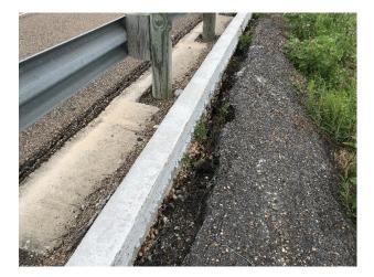
G11: MBGF Structure Rolling Over Due to Erosion – NBML North of FM 1847
