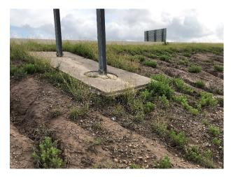
G6: Sign Foundation Exposed Due to Erosion – SBML North of RR Crossing No. 1
