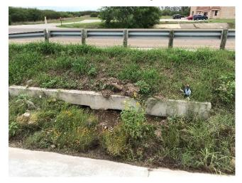
D6: Silt Accumulation at Culvert Crossing – NBFR North of Ditch No. 3
