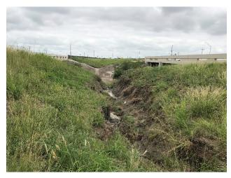
G15: Run Off Erosion Cutting Through Inside Median – Ditch No. 3
