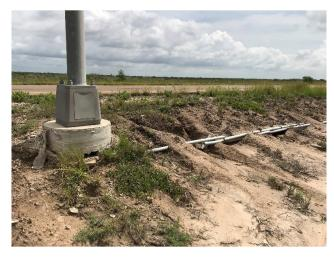
M1: Exposed Conduit/Foundation Due to Erosion – NBFR North of RR Crossing No. 1
