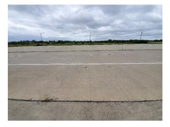
PV25: Transverse Cracking – SBML E of Entry Toll Gantry
