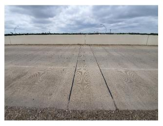
B7: Bridge Joint Requiring Resealing – SBML FM 3248 Bridge
