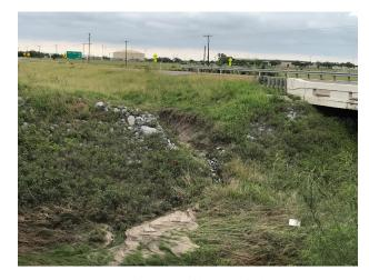
G10: Stone Rip Rap Failure - Ditch No. 3
