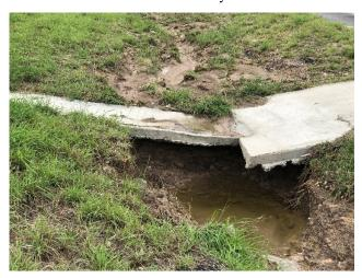
G14: Run Off Erosion Created Void Under Flume -NMBL North of RR Crossing No. 3
