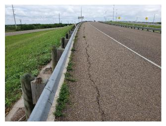
PV12: Crack in Asphalt - NBML W of RR Bridge
