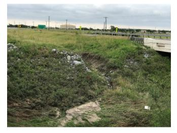
D5: Stone Rip Rap Failure – Ditch No. 3
