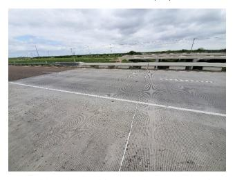
B19: Bridge Joint Requiring Resealing – SBML W of Ditch No. 3
