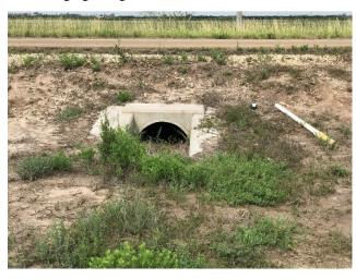
D1: Overgrown Vegetation/Silt Accumulation at Culver Crossing – SBML South of RR Crossing No. 1
