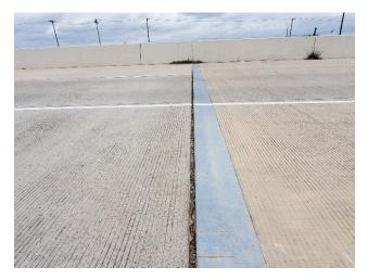
PV19: Joint Require Sealing and Cleaning – NBML East of Ditch No. 3
