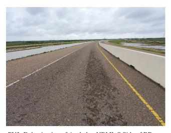
PV3: Delamination of Asphalt – NBML S Side of RR Bridge
