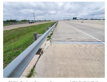
PV20: Broken Concrete Pavement – NBML Exit Toll Gantry
