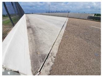
B16: Bridge Joint Requiring Resealing – NBML E Side of  $2^{nd}$  RR Bridge
