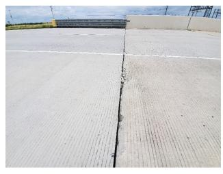
PV17: Damage Concrete at Approach of Gantry – NBML E of Old Alice Rd
