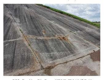
B25: Cracking Rip Rap – NBML FM 1847 Bridge
