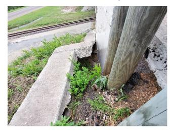
B17: Erosion Beneath Rip Rap – SBML W Side of 2nd RR Bridge
