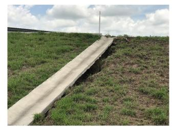
G16: Run Off Erosion Created Void Under Flume – SBML South of FM 1847
