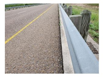
PV7: Separation of Asphalt and Mow Strip – NBML E of FM 1847
