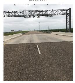
PM6: Faded Pavement Markings at Bridge – NMBL at Toll Gantry No. 2
