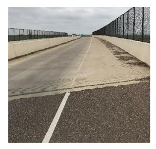
PM3: Faded Pavement Markings at Bridge – NBML South of RR Crossing No. 1
