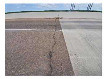
PV37: Cracking at Approach to Toll Gantry – SBML W of Exit Toll Gantry
