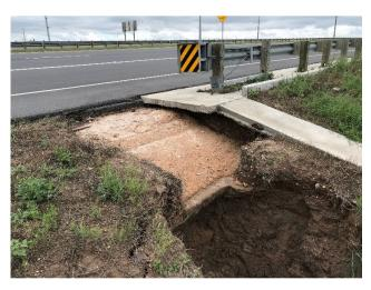
G9: Run Off Erosion at Front Slope With exposed Roadway Flex Base and Subgrade – SBML North of FM 1847
