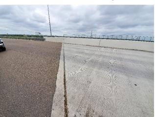
B14: Bridge Joint Requiring Cleaning and Resealing – SBML E Side of 2nd RR Bridge
