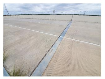
B21: Bridge Joint Requiring Cleaning and Resealing – SBML Old Alice Bridge
