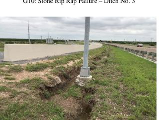
G13: Run Off Erosion Cutting Through Inside Median - NBML North of RR Crossing No. 3
