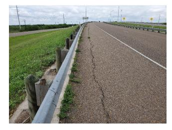
PV12: Crack in Asphalt - NBML W of RR Bridge
