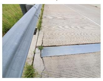
PV22: Broken Concrete Pavement – SBML Entry Toll Gantry
