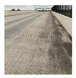
PM5: Faded Pavement Markings at Bridge Approach – NBML South of RR Crossing No. 1
