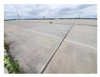
B22: Bridge Joint Requiring Cleaning and Resealing – SBML Old Alice Bridge
