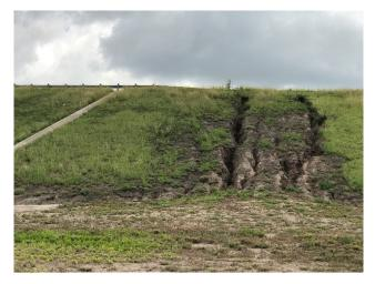
G17: Run Off Erosion Caused by Ineffective Flume – NBML North of FM 1847
