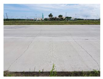
PV28: Transverse Cracking – SBML E of Ditch No. 3
