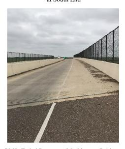
PM3: Faded Pavement Markings at Bridge – NBML South of RR Crossing No. 1
