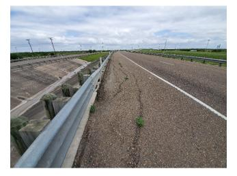
PV13: Cracks in Asphalt – NBML E of Ditch No. 3
