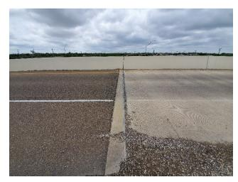
B5: Bridge Joint Requiring Cleaning and Resealing – SBML E Side of FM 3248
