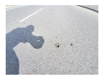
PV30: Pothole in Asphalt – SBML W of RR Bridge
