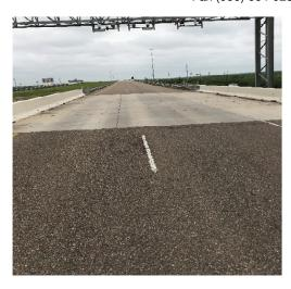
PM6: Faded Pavement Markings at Bridge – NMBL at Toll Gantry No. 2
