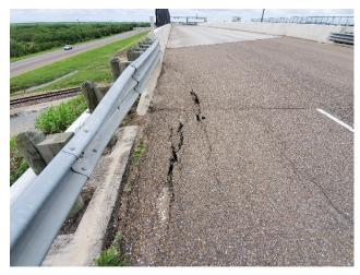
PV11: Cracks in Asphalt – NBML W of RR Bridge
