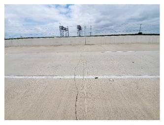
PV16: Transverse Cracking – NBML E of Old Alice
