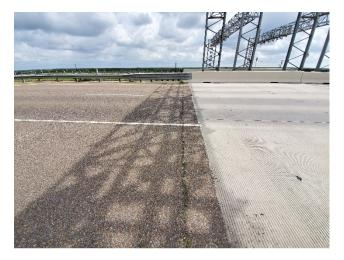
PV31 Cracking at Approach to Toll Gantry – SBML W of Toll Gantry
