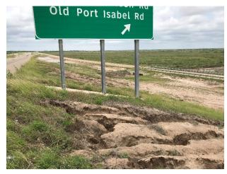
G4: Run Off Erosion at Front Slopes – NBML North of RR Crossing No. 1
