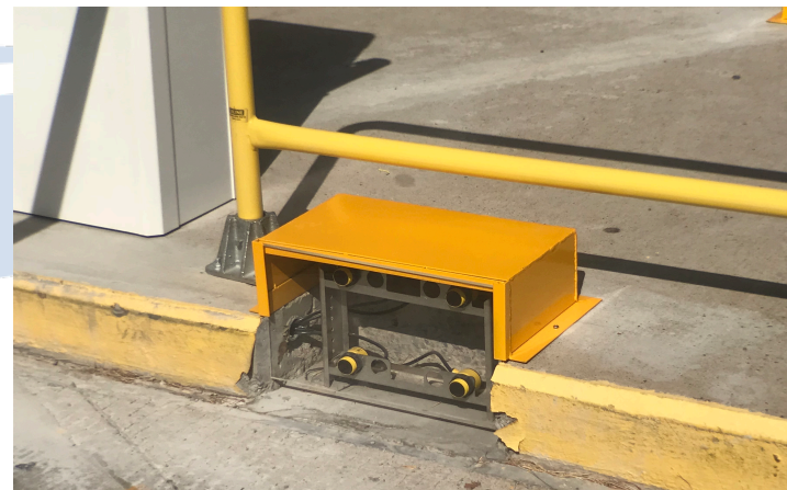
Figure 5 Photo Cell Technology for axle detection
