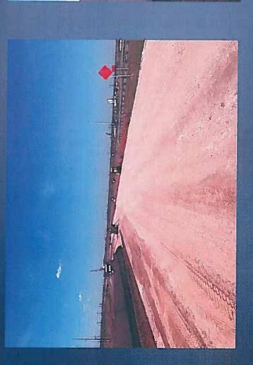
PLACING GEOGRID AND FLEXBASE – SOUTH BOUND (RAMP SECTION) FACING WEST
