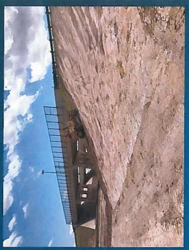
INSTALLING METAL GUARD FENCE AT BRIDGE (FACING EAST)
